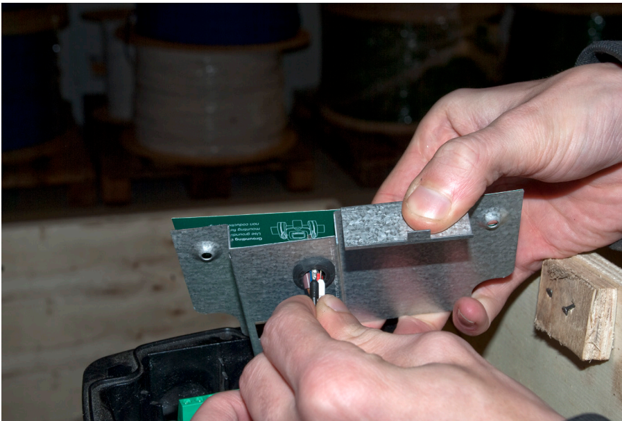
8. Lead cables in the metal cover plate
